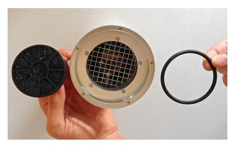
2. Discard the old filter cartridge and insert the new cartridge. The o-ring will easily snap into place and secure the filter.
