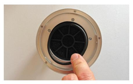
3. The o-ring will bend until it fully snaps into its groove to retain the filter cartridge.
